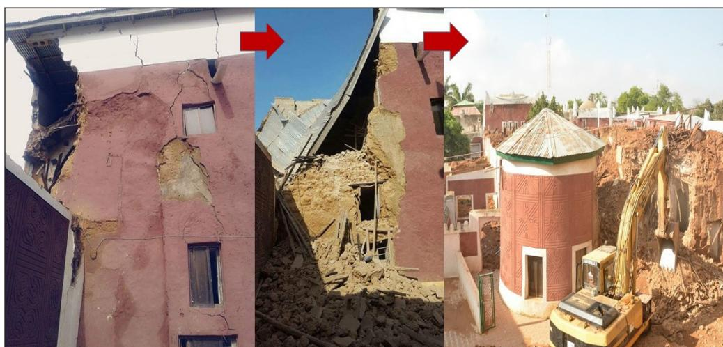
Figure 8. The Emir's wing self-collapse and demolition process after attaining ageing and limit of repair
