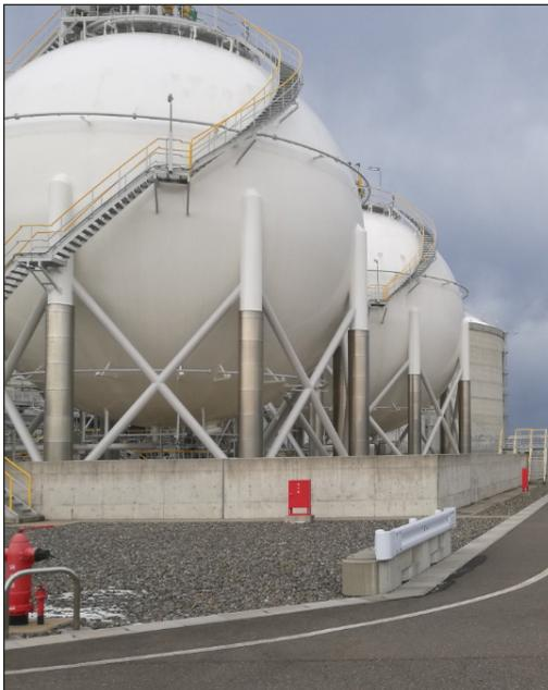
Figure 6. INPEX LNG regasification terminal - bund around LPG sphere
