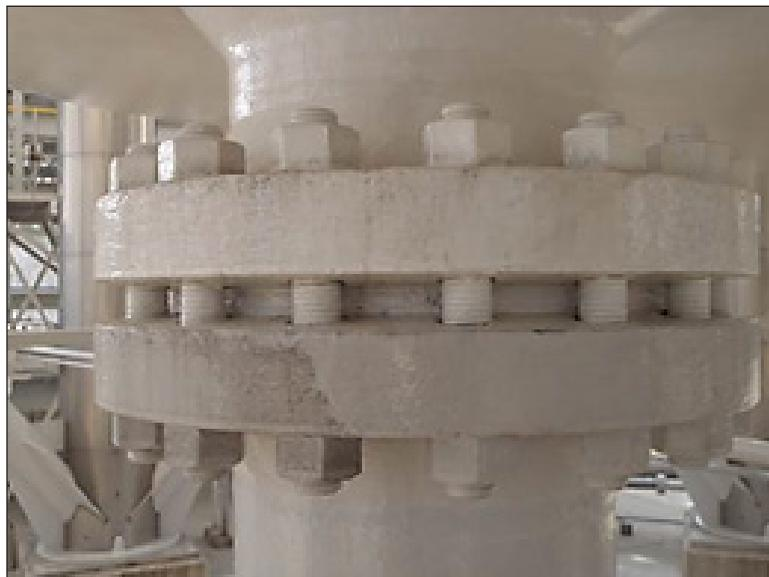
Figure 4. INPEX LNG regasification terminal - Non-leak flange
