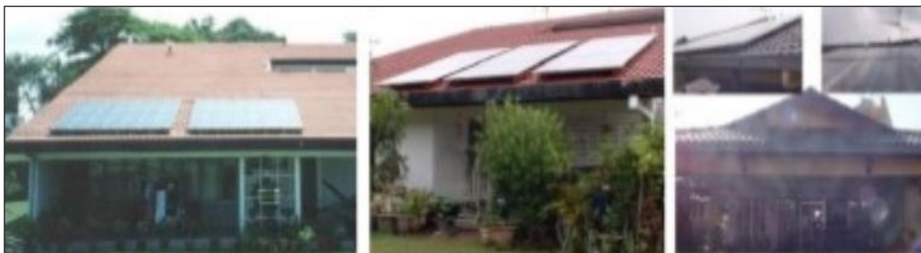
Figure 1. Port Dickson, Shah Alam and Subang Jaya first home installed BIPV (Haris et al., 2003)
